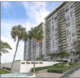
The Charter Club, Miami Building Recertification & Deck Repairs
