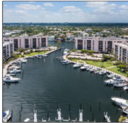
Yacht & Racquet Club of Boca Raton Structural Integrity Reserve Study
