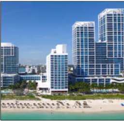
Carillon Hotel, Miami Storm Damage Assessment
