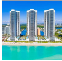
Trump Tower II, Miami Façade Restoration and Paint
