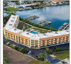
Hickory Harbor, Naples Storm Damage Assessment
