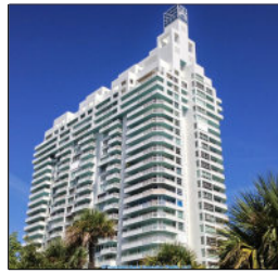
Southpointe Tower I, Miami Milestone Inspection Survey
