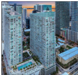
Axis on Brickell, Miami Façade Restoration and Paint
