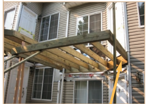
Deck ledger to rim joist connection.
